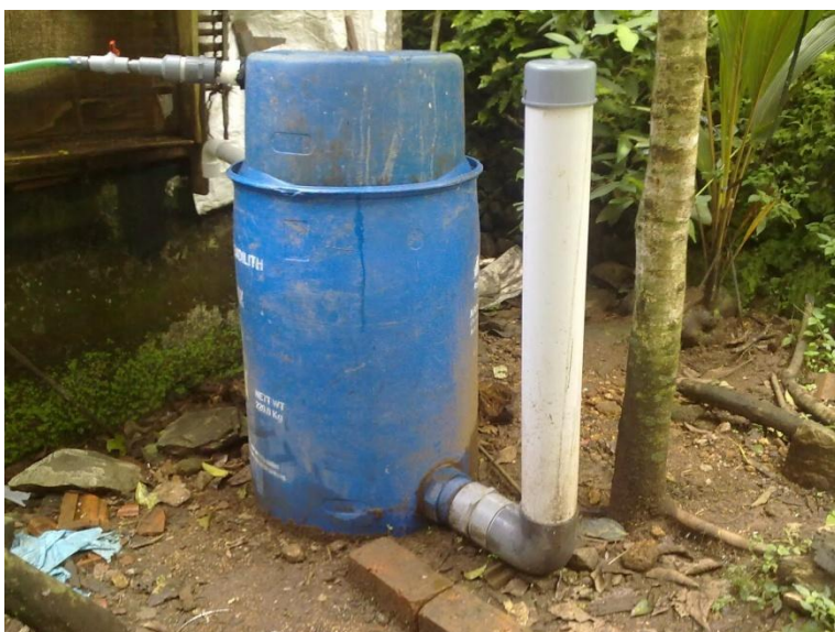
Figure 28: home made digester with PVC tube as inlet and outel pipe, source: http://myhomehobbies.blogspot.ch/2011/09/home-made-bio-gas-plant.html
