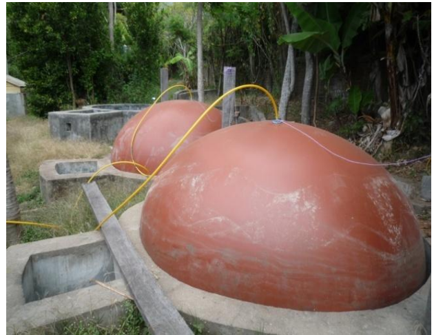
Figure 11: Digester full after 10 days without using biogas
