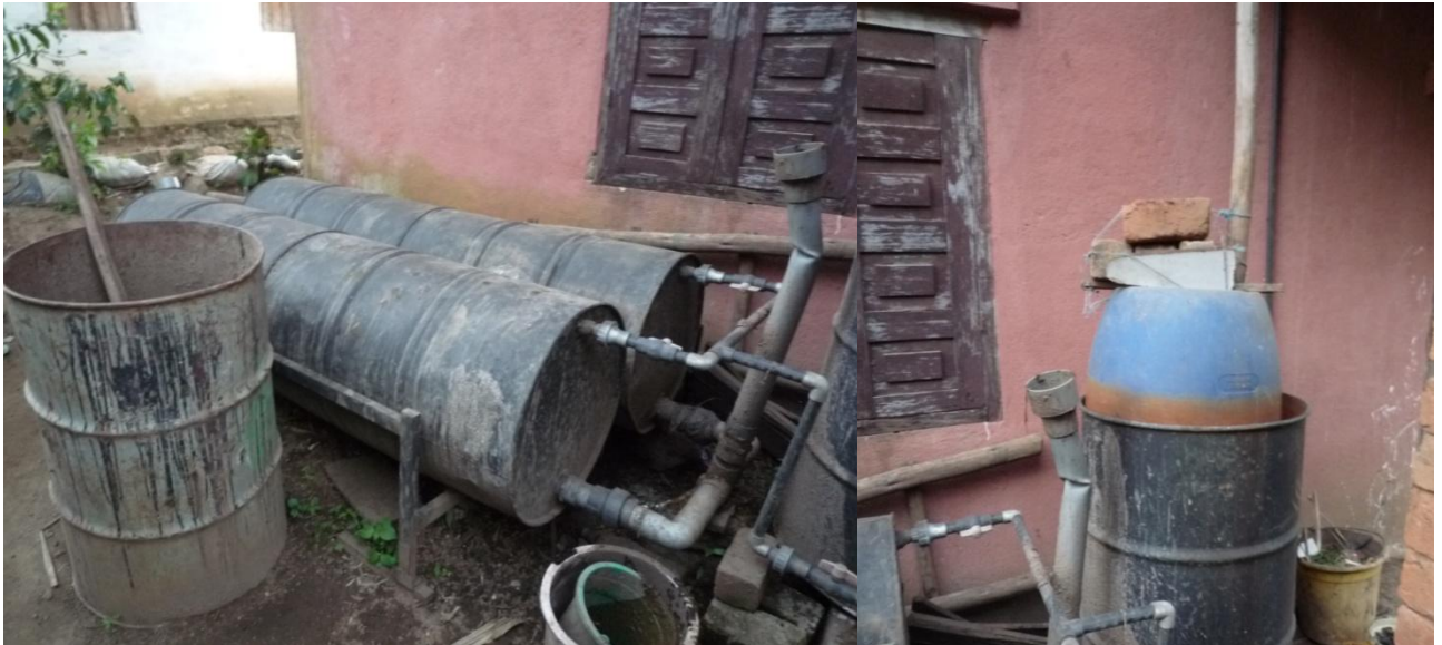
Figure 25: "home made" 1m3 plant implemented by an NGO. It is not sufficient for the daily needs of the only women using it.
