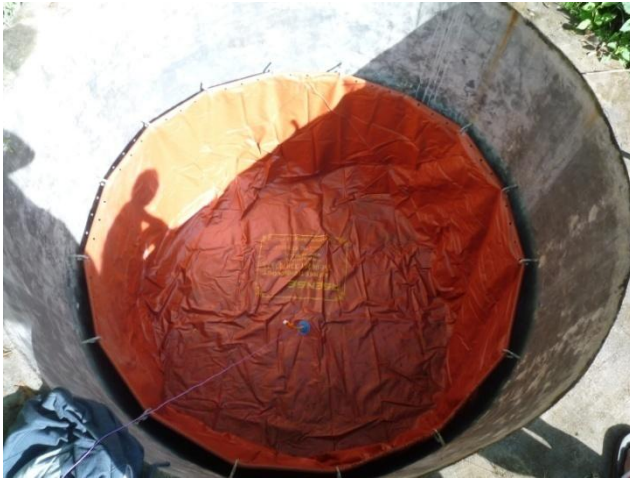
Figure 6: installation of the tarp
